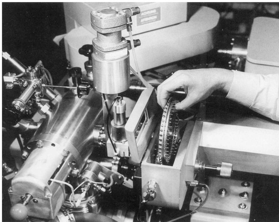
**Fig. 5.12** Finnigan MAT AUDEVAP system where the turret wheel with 46 crucibles is being inserted into its housing. The probe mechanism is to the *right*, the vacuum lock and the ion source housing to the *left*. The mass spectrometer may either be a Finnigan MAT 212 or MAT 311 double-focusing sector instrument of BE geometry (Reproduced from Finnigan MAT technical documentation by courtesy of Thermo Fisher Scientific)
