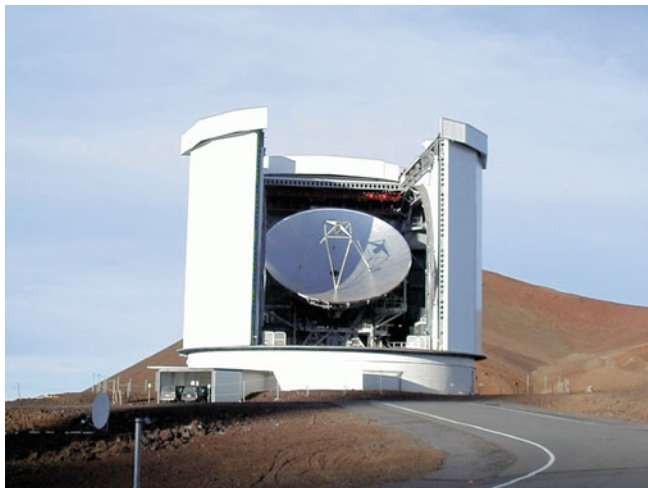
Fig. 1.28 Left: The James Clerk Maxwell Telescope (JCMT) on Mauna Kea has a 15 m dish. It is protected by the largest single piece of Gore-Tex, which has a transmissivity of 97 % at sub-millimeter wavelengths. Right: The Atacama Pathfinder Experiment (APEX) 12-m sub-millimeter telescope has been in operation since 2005. It is located
